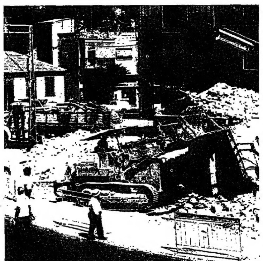
HISTORY LESSON. — A bulldozer yesterday demolishing the house in which Petah Tikva's first settlers lived, at the Mayor's orders. The building, known to oldtimers as the Lachman House, served the early settlers as a fort during the periodic Beduin attacks and was later used as a winery. The demolition order was given in order to widen Rehov Haim Ozer, on which the house stood until yesterday. (Dekal)
